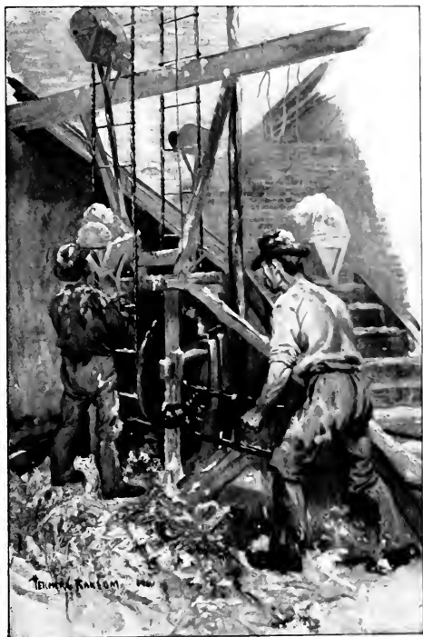
Endless Chain Hod Elevator in Use in America.
